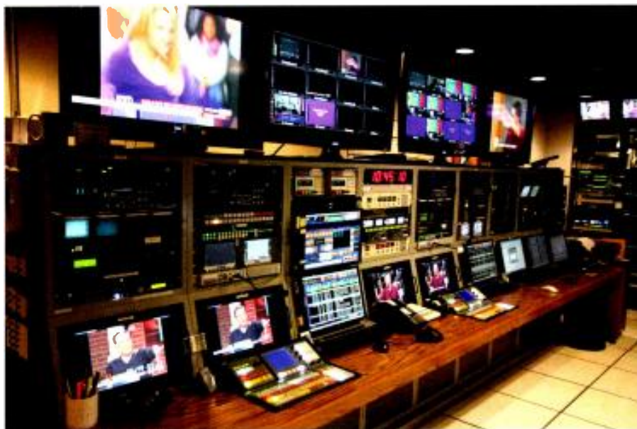
WDRB selected a UTAH-400/144 digital routing switcher to support its transition to HD news production. The 9RU switcher offers crosspoint redundancy and signal presence detectors on all inputs and outputs.
